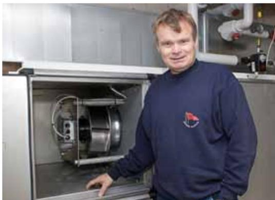
*Significant savings can always be achieved by switching from belt-driven AC fans to modern EC technology.*
